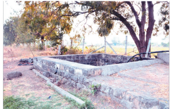
Photograph No 2–Scene of crime showing well having parapet wall.
