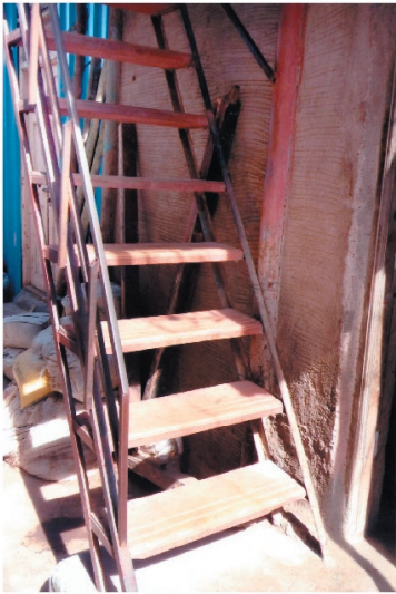
Photograph no 4 - Wooden staircase with iron railings at the entrance of door.
